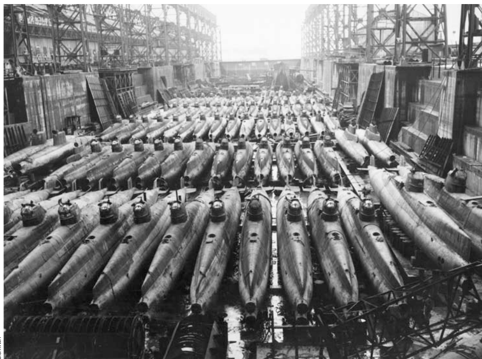
A SPENT FORCE? The commonly held view is that Japanese industry was practically nonexistent by the summer of 1945. But as this photo of midget submarines at the Kure naval base taken shortly after the Japanese surrender shows, highly technical priority items not only could still be produced in quantity by the Japanese but also could be missed or successfully hidden from the prying eyes of U.S. reconnaissance aircraft for nearly six months after they commenced operations from nearby Okinawa.
